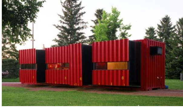
Figura 3 - Vista externa do Mobile Dwelling Unit
